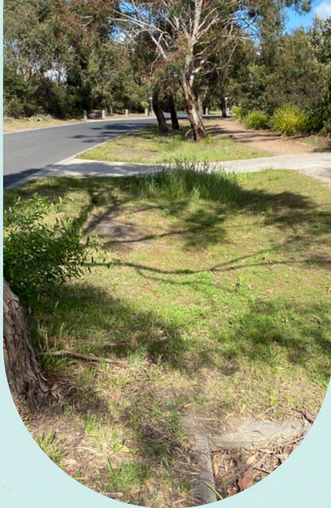
Road shoulders can be softened with low edges to grassed swales
